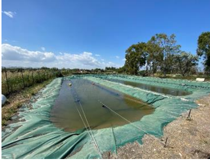
Open-circuit underground basins for biological species maintenance at CNR IRBIM Lesina
